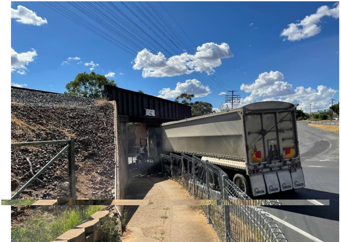
Figure 2-13: Heavy vehicle traversing underpass
