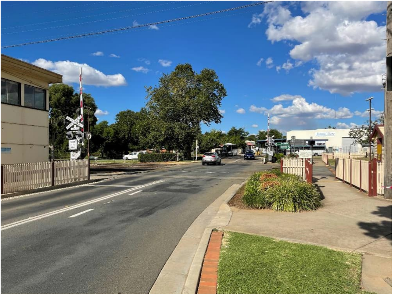
Figure 2-10: Level crossing, looking east toward Main Street
