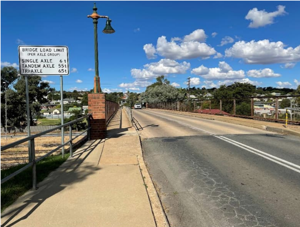
Figure 4-4: Kemp Street Bridge (looking east)
