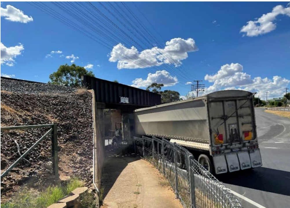
Figure 4-8: Olympic Highway underpass (looking west)
