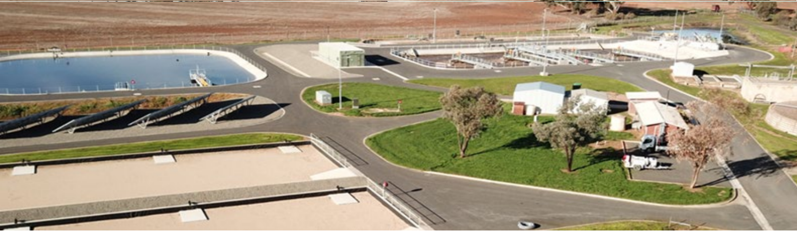
Junee Sewage Treatment Plant
