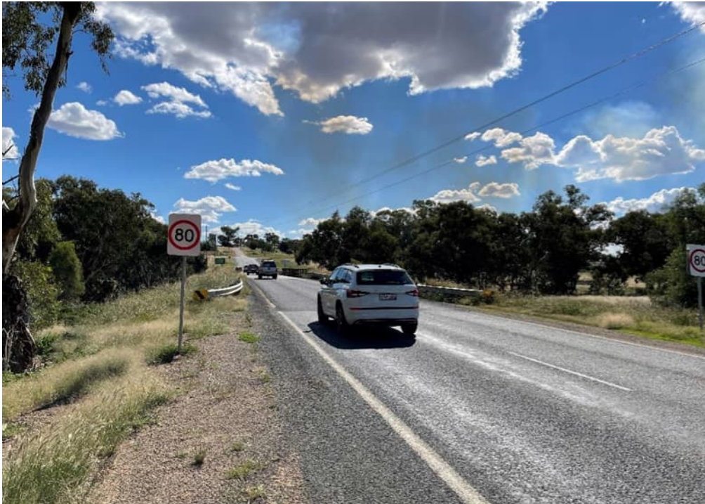
Figure 4-7: HL Robinson Bridge (looking west)
