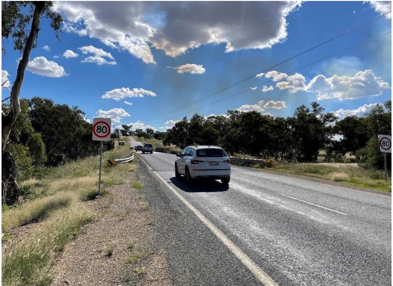
Figure 2-16: HL Robinson Bridge, with intersection of Old Junee Road and Goldfields Way in background
