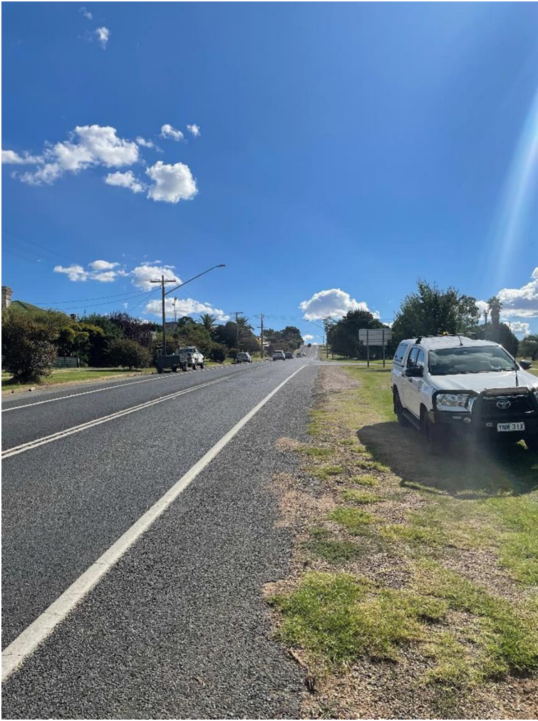
Figure 4-9: Olympic Highway west of Kemp Street intersection (looking west)
