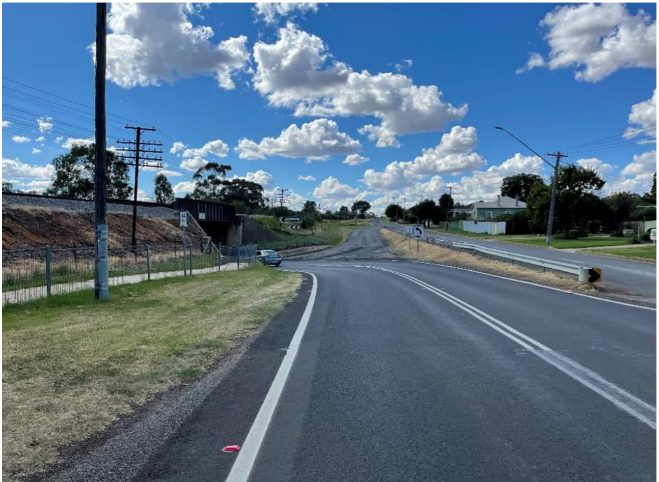
Figure 2-12: Northbound approach to rail underpass
