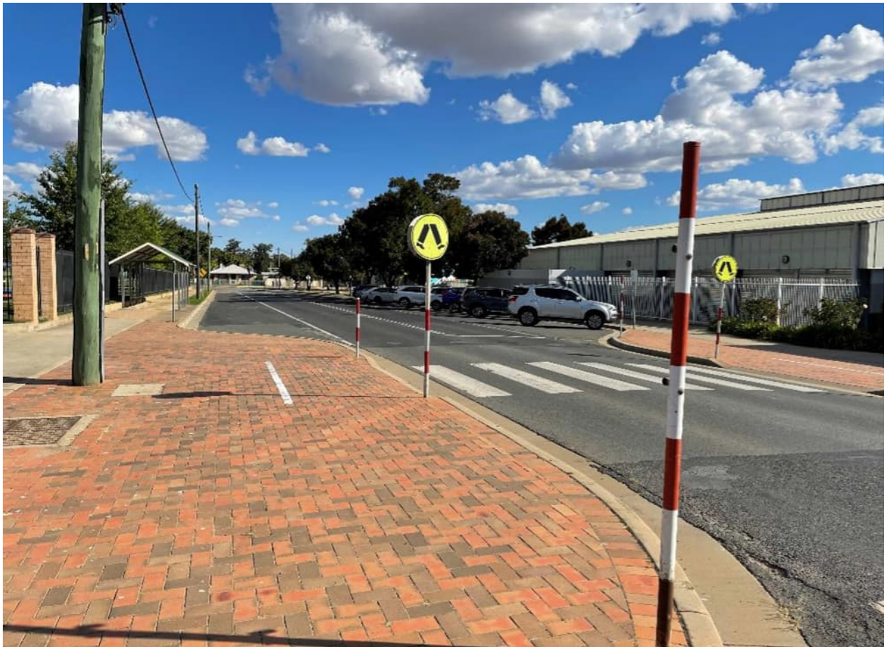
Figure 2-17: Zebra Crossing over Lorne Street, looking south toward school bus stop
