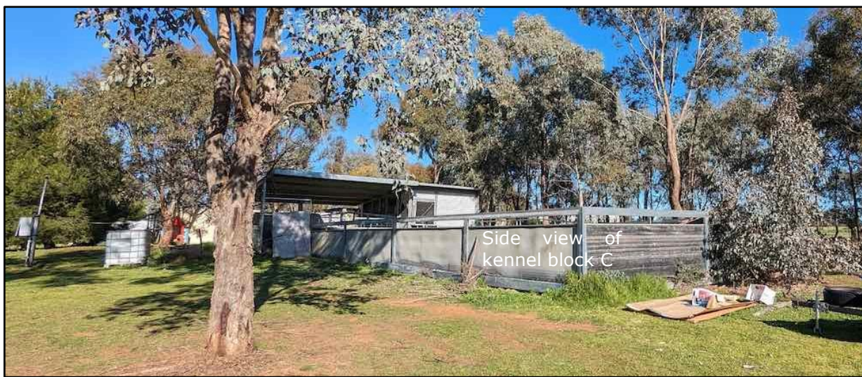
Figure 10: Side view of kennel block C (Source: SP 2023)
