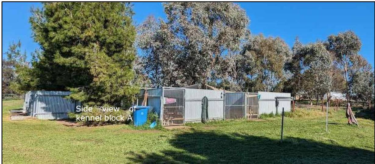
Figure 8: Side view of kennel block A (Source: SP 2023)
