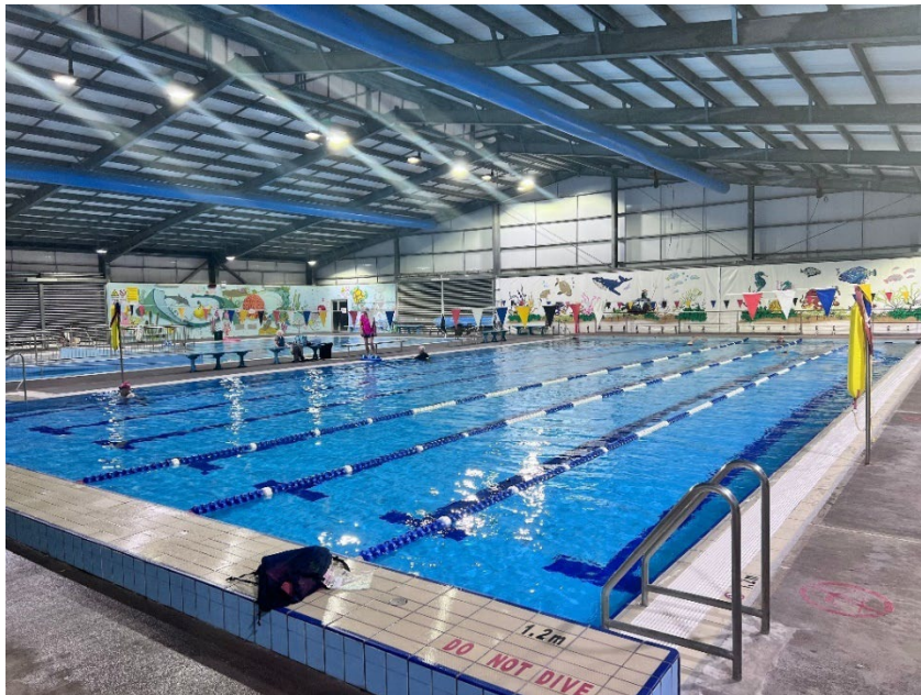
Photo: Swimming Pool Re Titling Project at Junee Recreation and Aquatic Centre.
