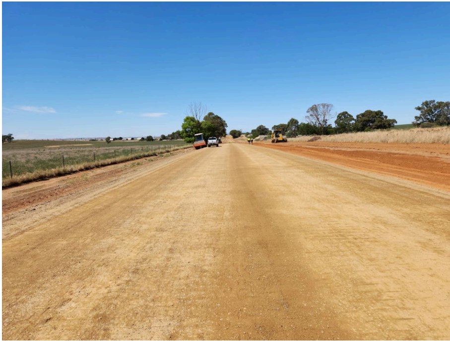
Photo: Road Construction.
