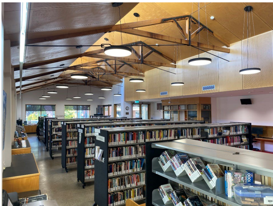
Photo: Library light refurbishment.
