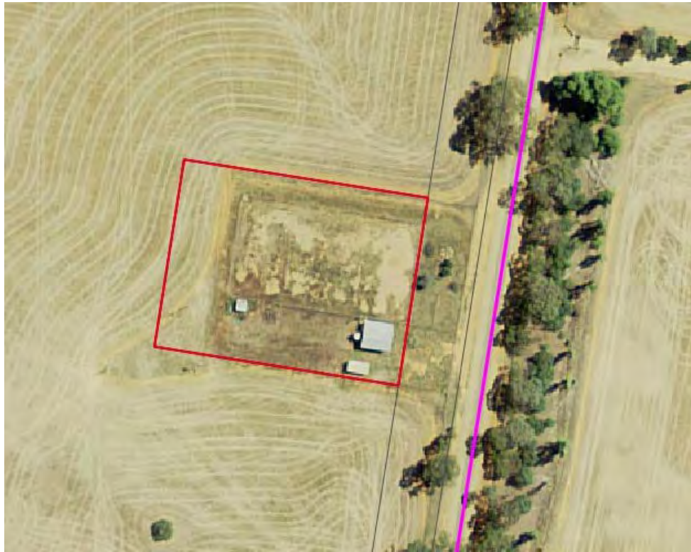
Figure 1 - Infrastructure at CPT&CC Facility
